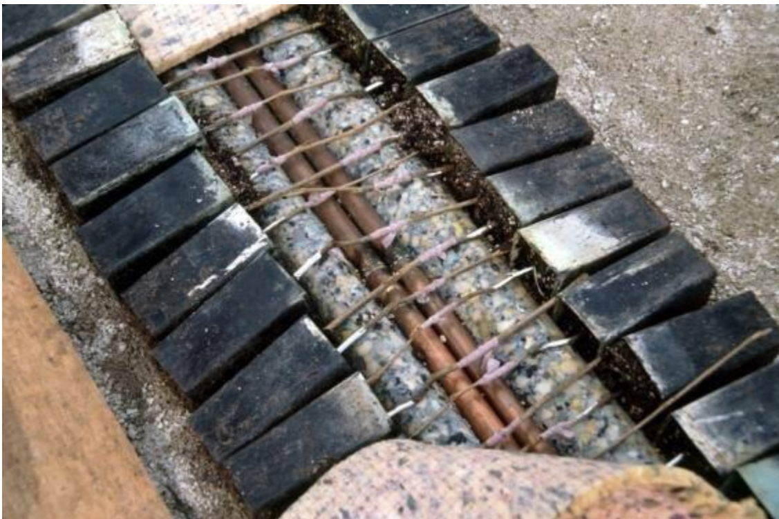
Top view photo of a hot-pipe system keeping rows of grafts warm.
